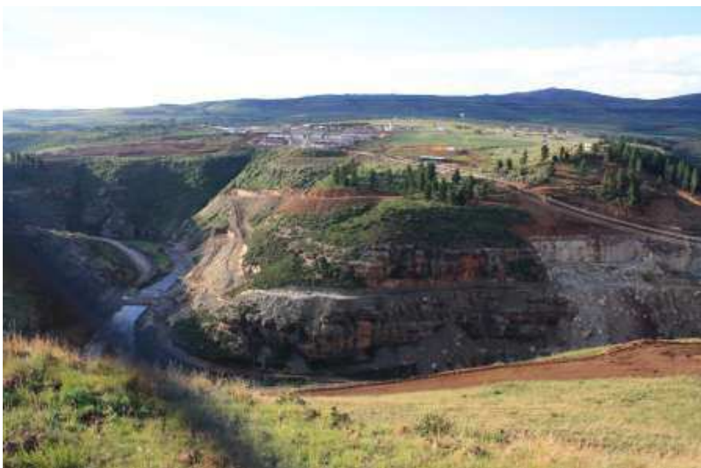
Metolong Dam under construction
