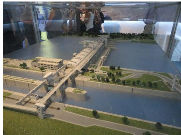
Model of Verbund Hydropower installation
